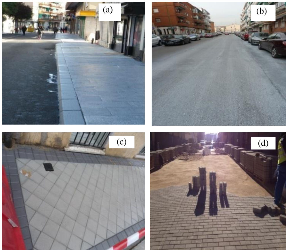
Figure 1. 13 (a) Photocatalytic sprays on sidewalk tiles, (b) draining bituminous pavements percolated with photocatalytic slurry, (c) photocatalytic tiles to pavement sidewalks, and (d) photocatalytic tiles to pavement roadways.
