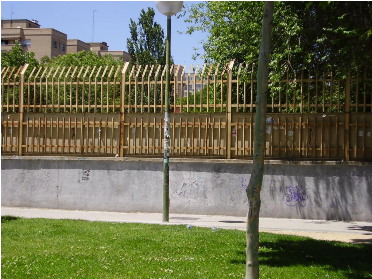
Figure 14: Exterior side of school wall (May 2009)
