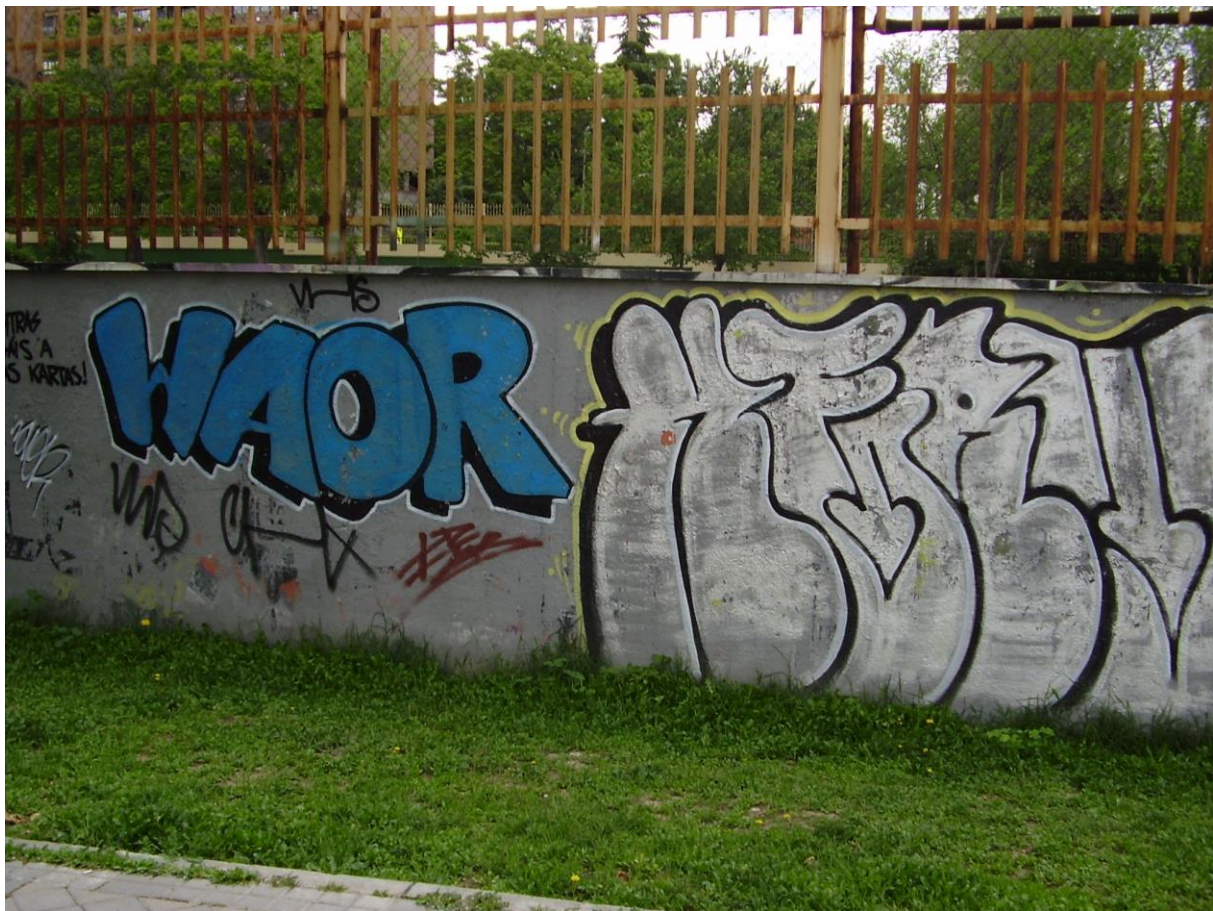
Figure 12: Exterior-side of school wall (2007-08 school year)
